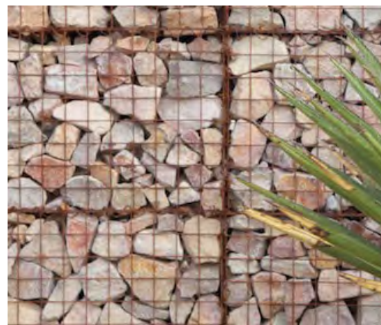
ROCK FILLED METAL CAGE @ COURTYARD
